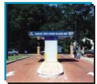
Drive-up Double Turn Kiosk, Canopy
