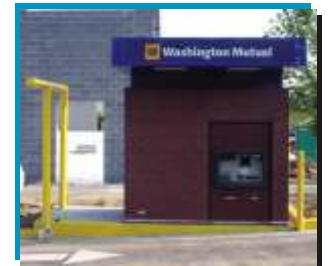
Drive-up Turn Kiosk, Canopy, and Custom Brick Exterior
