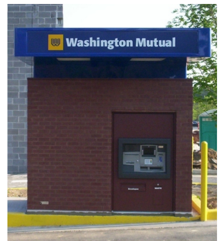
Turn Kiosk with Brick Exterior
