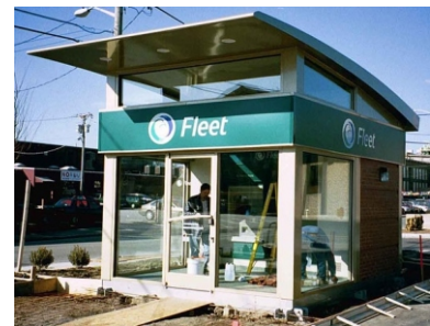
Installation of a Couvrette Lobby-style Classic Kiosk
