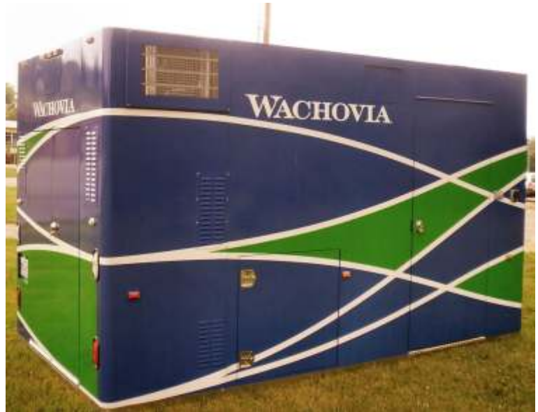
View of the Kiosk Entry access door.
