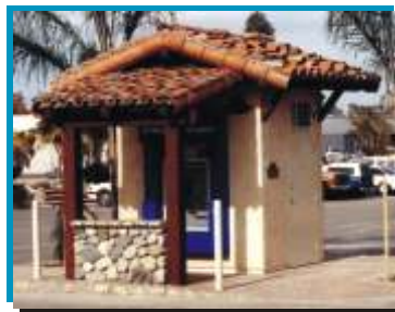
Classic Kiosk with Stucco Exterior and Spanish Tile Roof
